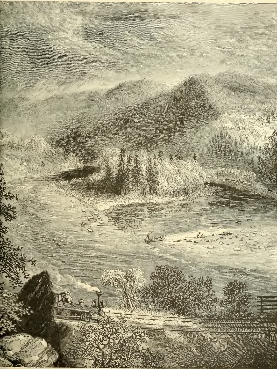
ROCK RIFT ON THE DELAWARE DIVISION ERIE RAILWAY, NEAR PORT JERVIS, N. Y.
